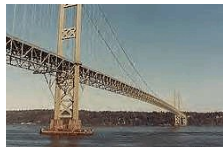
Tacoma Narrows Bridge (pre 2007)
